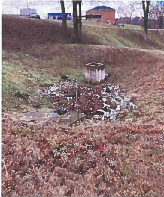
Detention Pond Entrance
