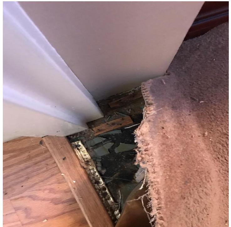
Blue 9x9 Floor Tile Under Carpet Room 0116 Sample 1-5
