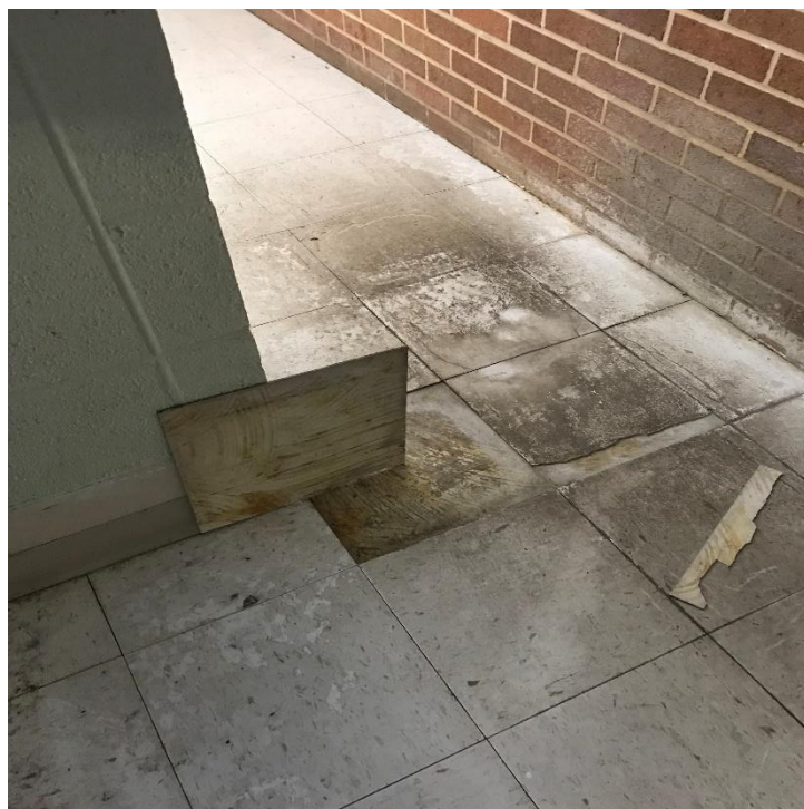
Off White Speckled 12x12 Floor Tile Room 0110 Sample 1-3
