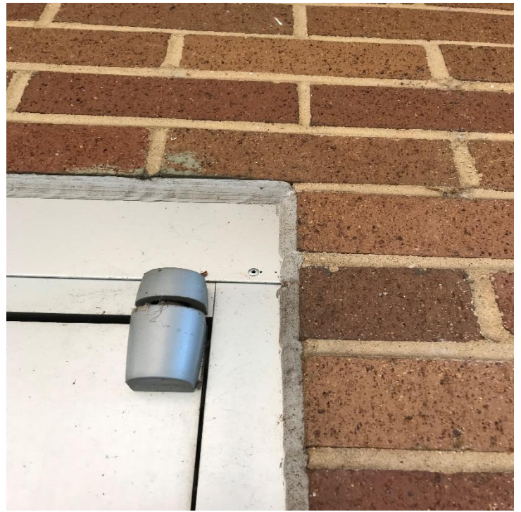
North Exterior Door Caulk Sample 2-9
