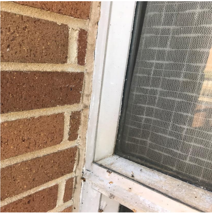
Exterior Window Caulk Northeast Sample 2-11
