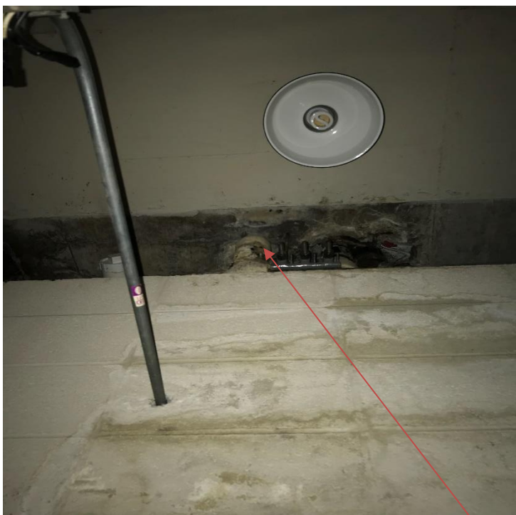
Elbow Insulation Room 0120 Sample 1-7
