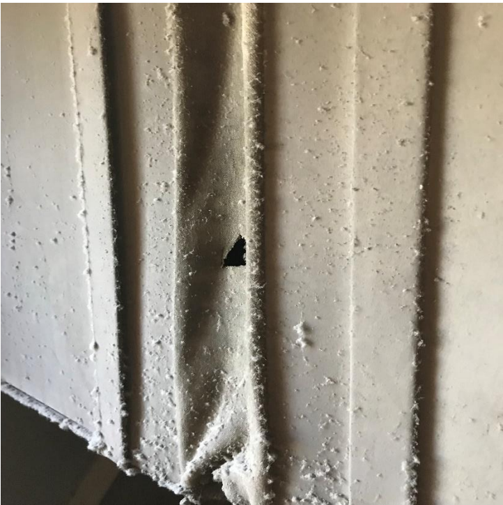
HVAC Vibration Dampener Room 0427 Sample 4-10
