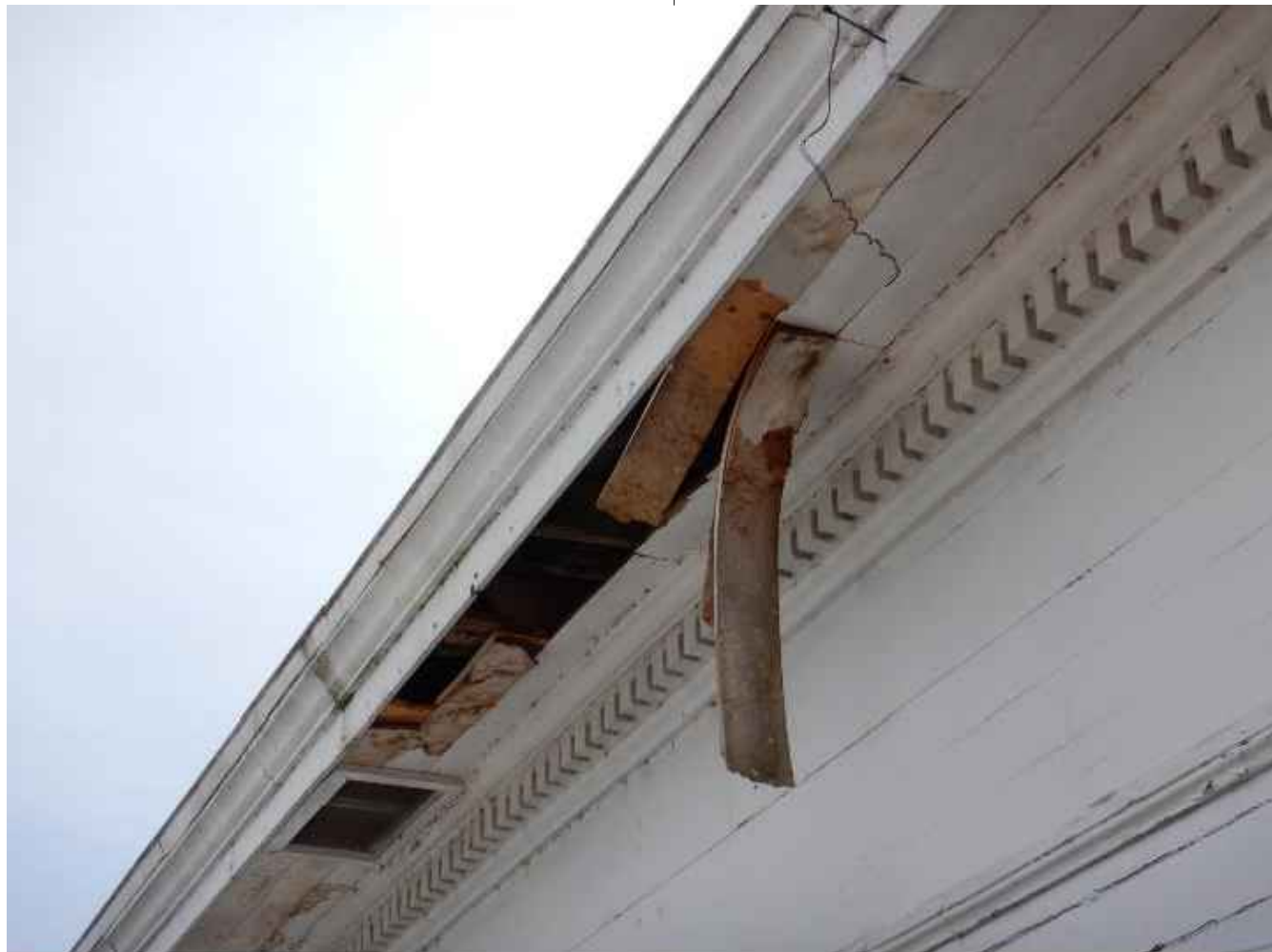
DAMAGED SOFFIT PANELING
