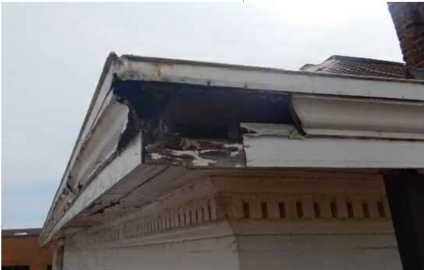
DAMAGED WOOD FASCIA/CORNICE
