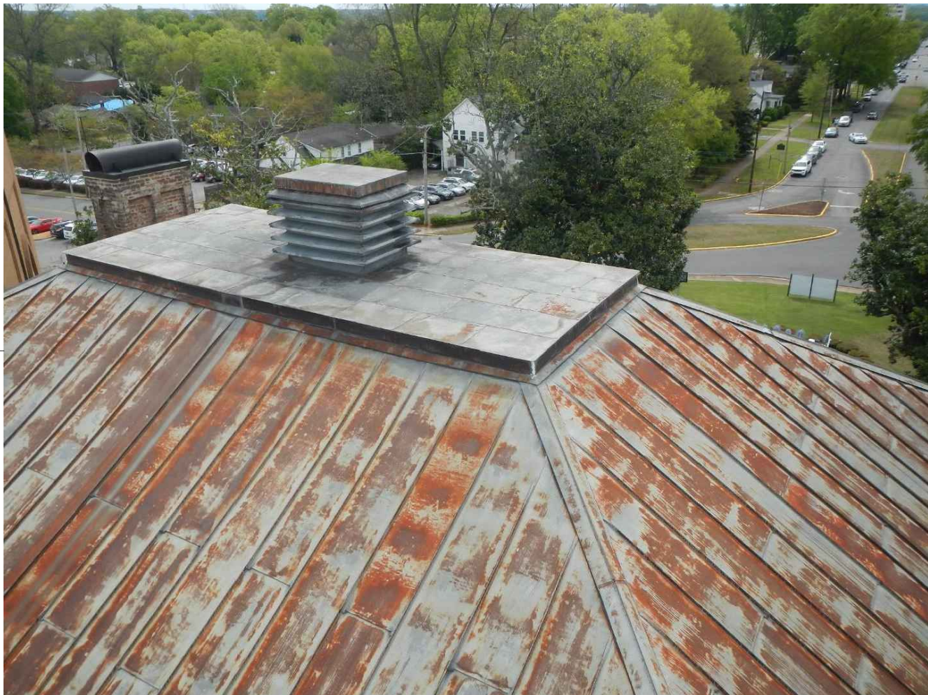
ROOF CORROSION PANELS
