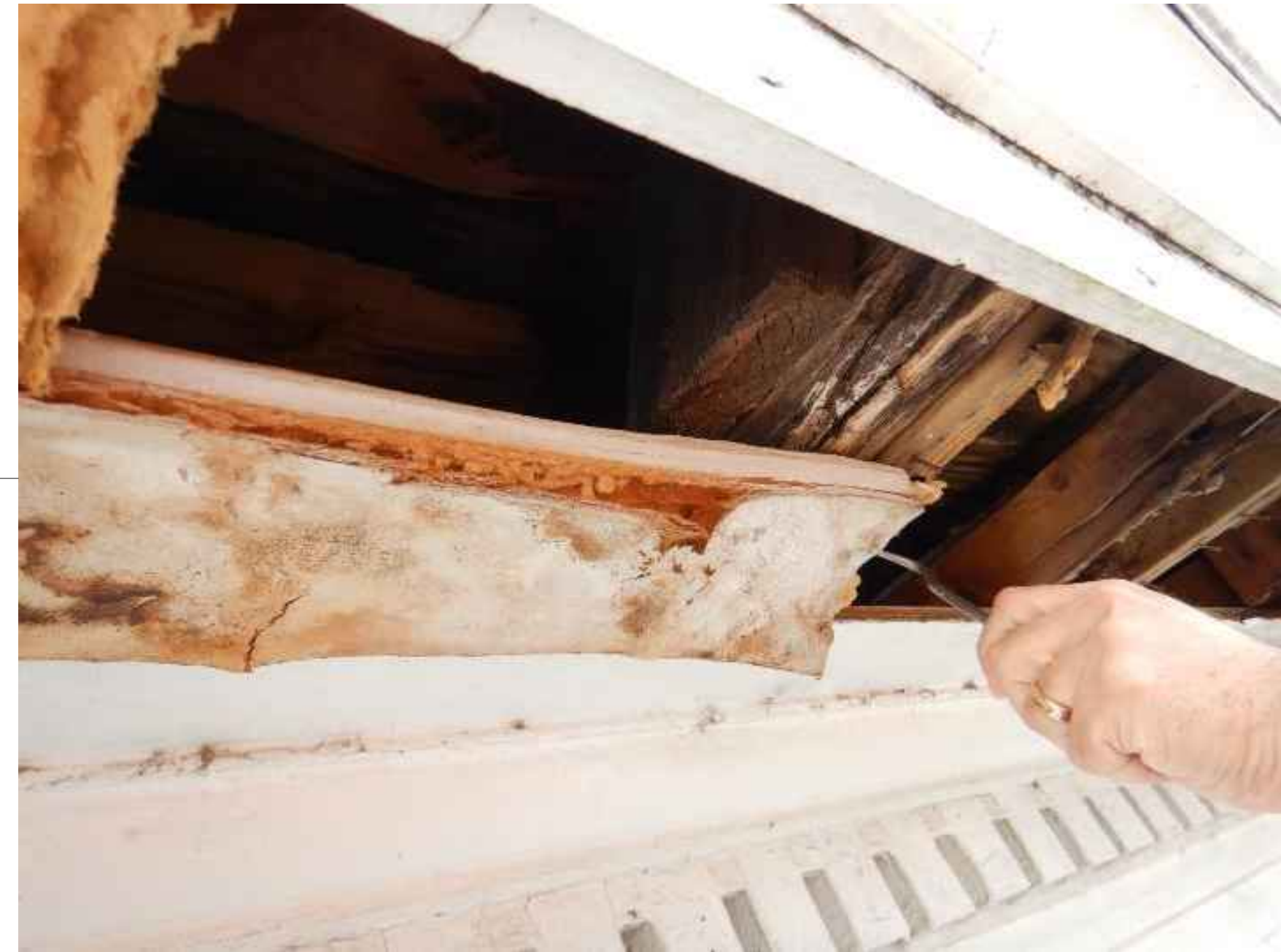
CORNICE GUTTER FRAMING SUPPORT Repair/replace all damaged cornice gutter framing support
