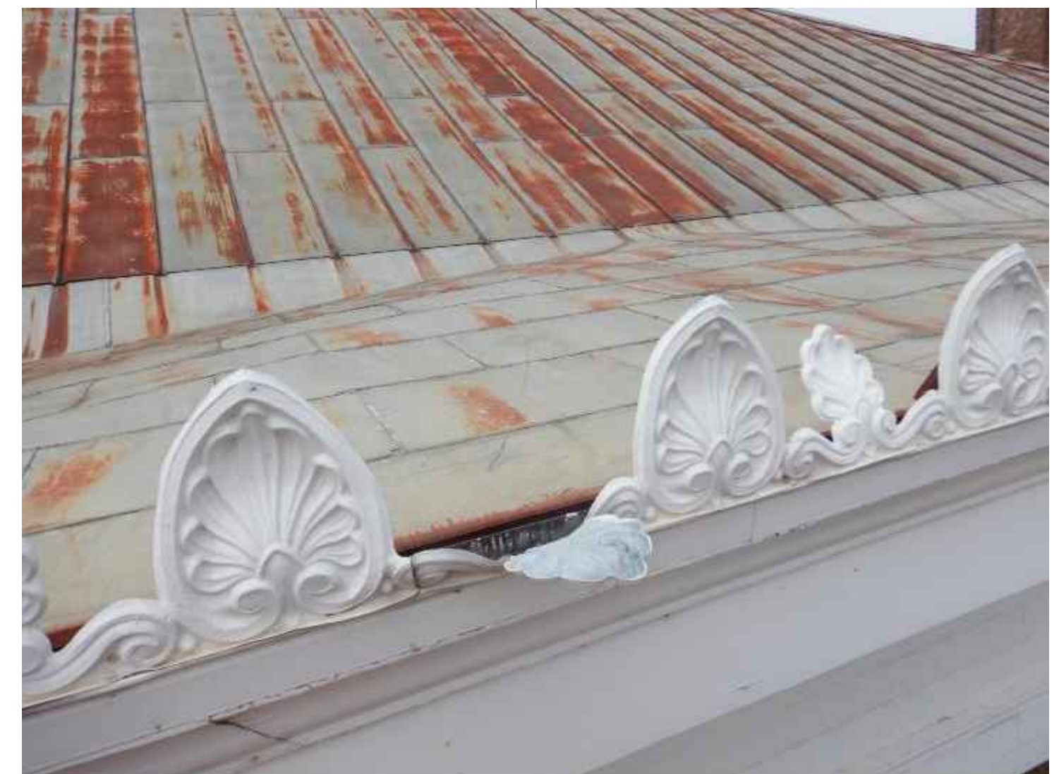
DECORATIVE SHEET METAL ELEMENTS Repair decorative sheet metal elements, secure and waterproof support frame.
