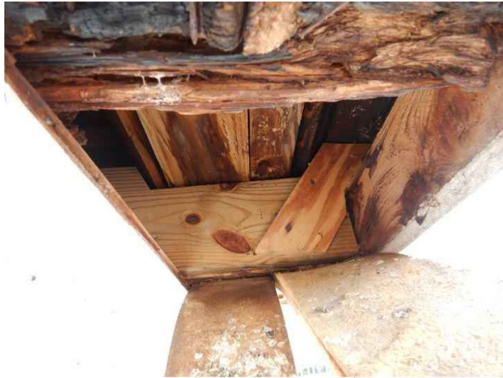
CORNICE GUTTER FRAMING Repair/replace all damaged cornice gutter framing
